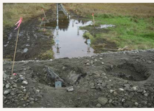
Installation of helical piers
