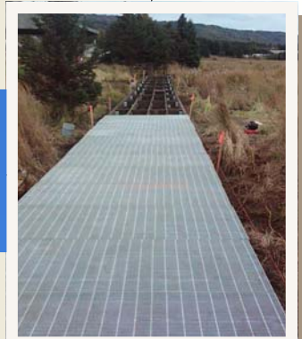
Grated galvanized steel trail surface in place
